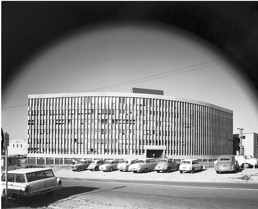
Figure 2: J D Story Administration building, UQ St Lucia (1966, Public Domain)
